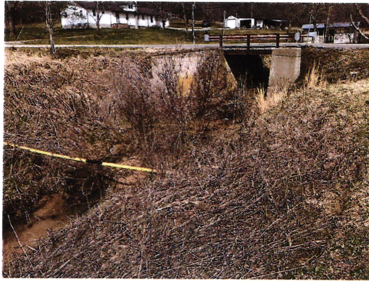
Photo 7 - Looking North/upstream at outlet, with exposed gas line shown
